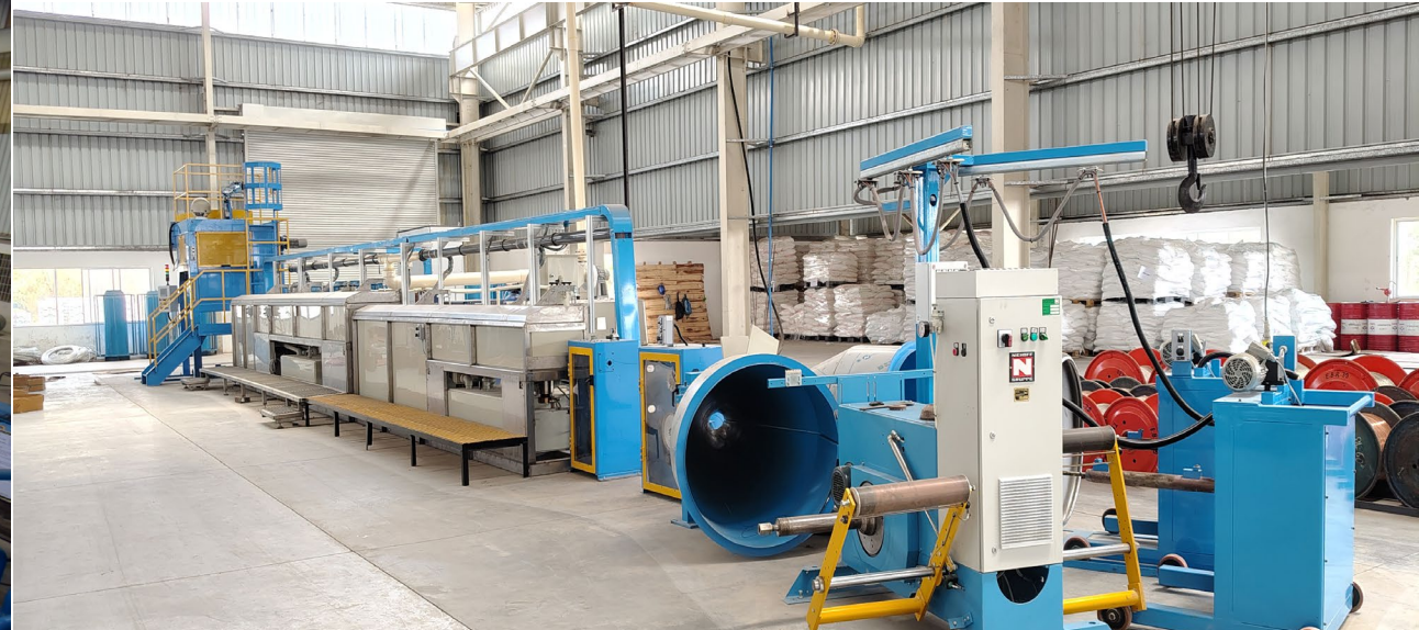
Elastomeric cables facility at Vadodara, Gujarat
