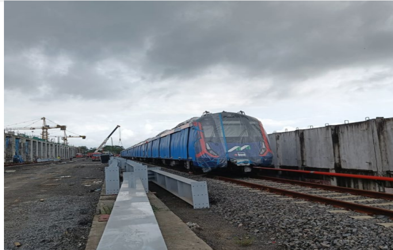
Track works, Mumbai Metro
