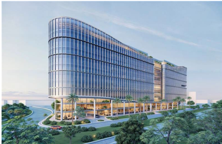
Commercial Building (Civil)
