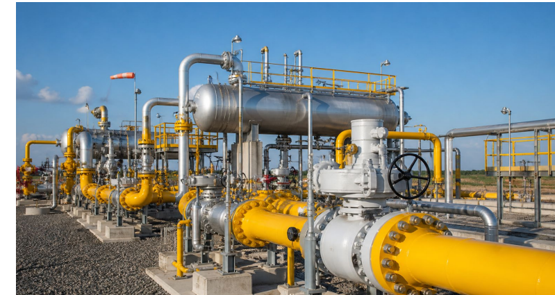
International - Composite Station Works (Oil & Gas)
