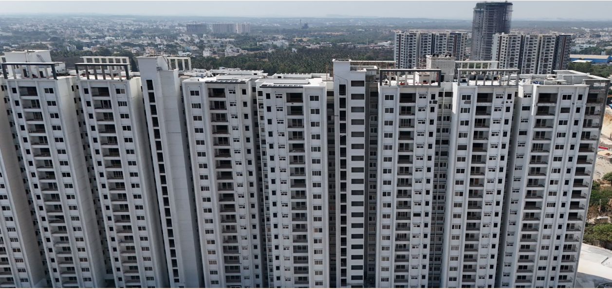
High Rise Residential Building, Bangalore, Karnataka
